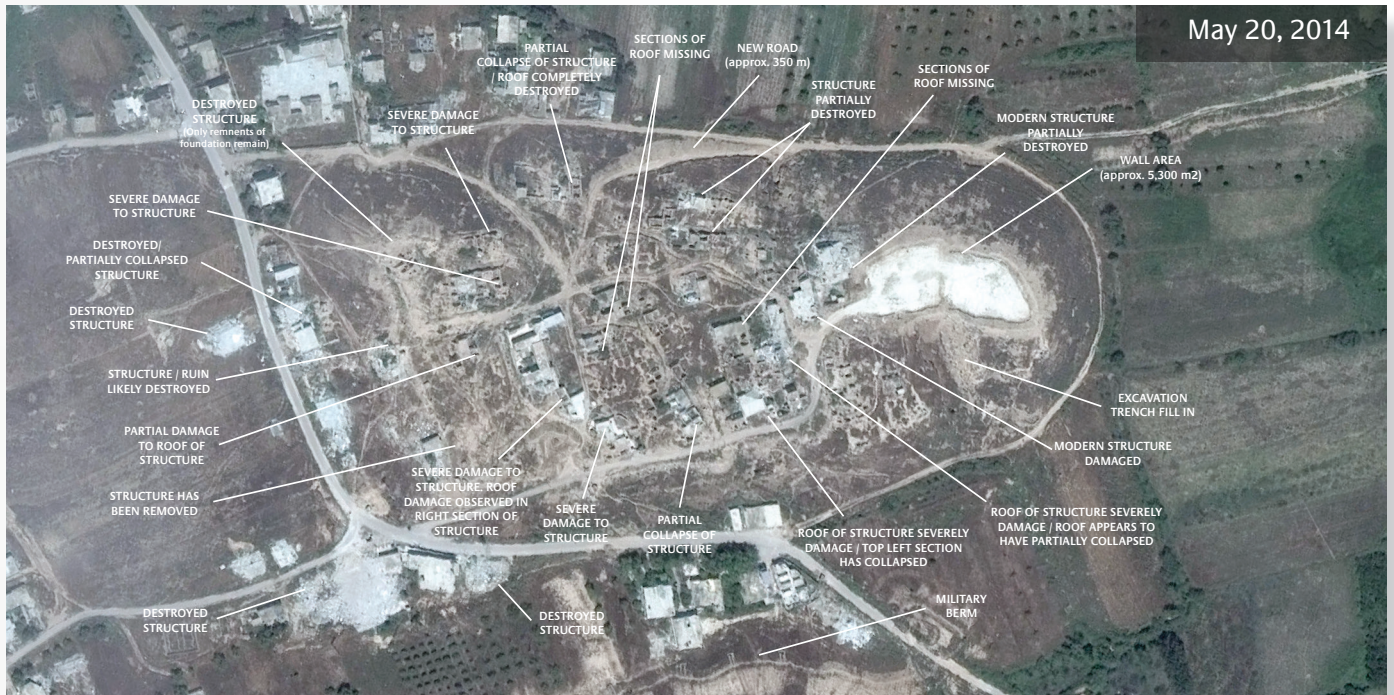
FIGURE 78. Extensive damage to Qadesh.
